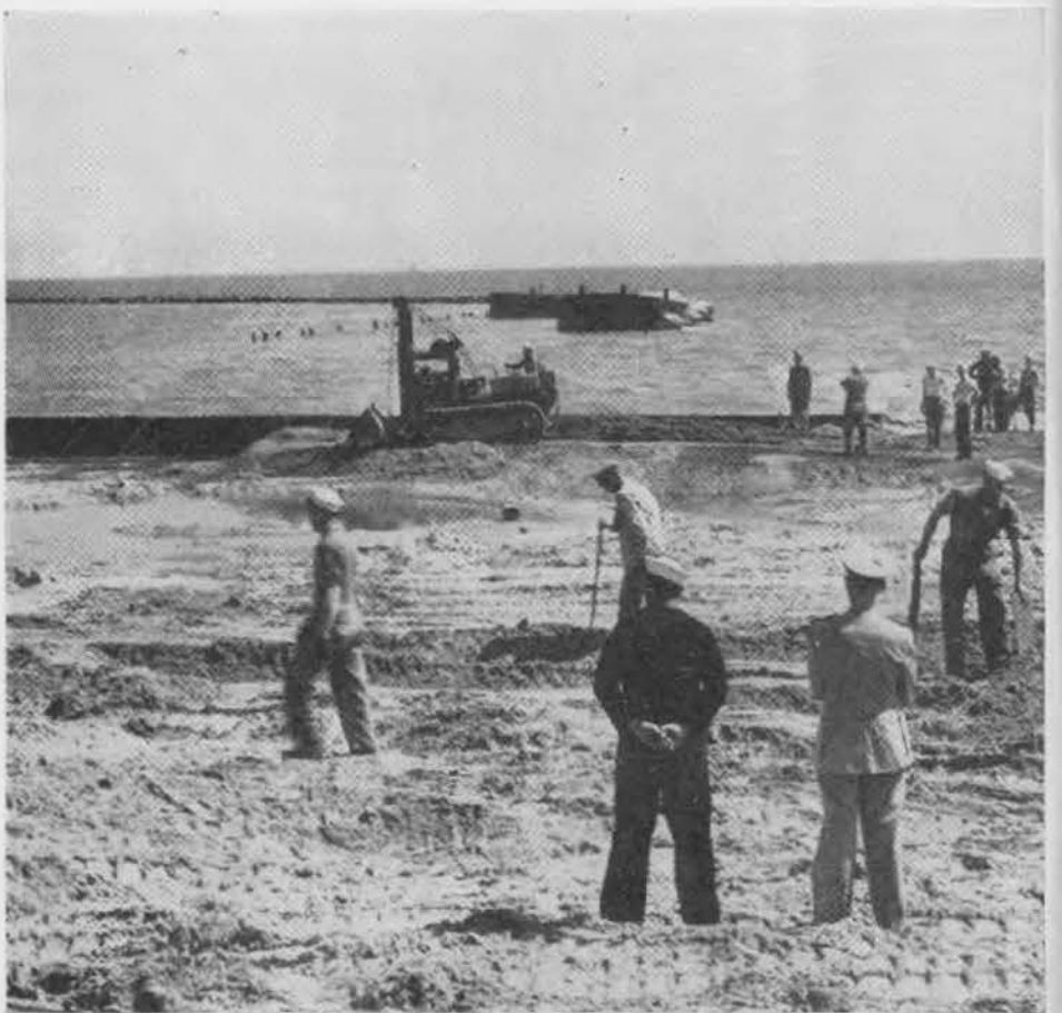
CONSTRUCTION TRAINING was also a part of our curriculum during our residence at A.B.D. Here, men of B. Company are making a fill on the Pontoon Launching Quay Project at the West Pier. In the foreground stand two critical inspectors from the Construction Training Department.
