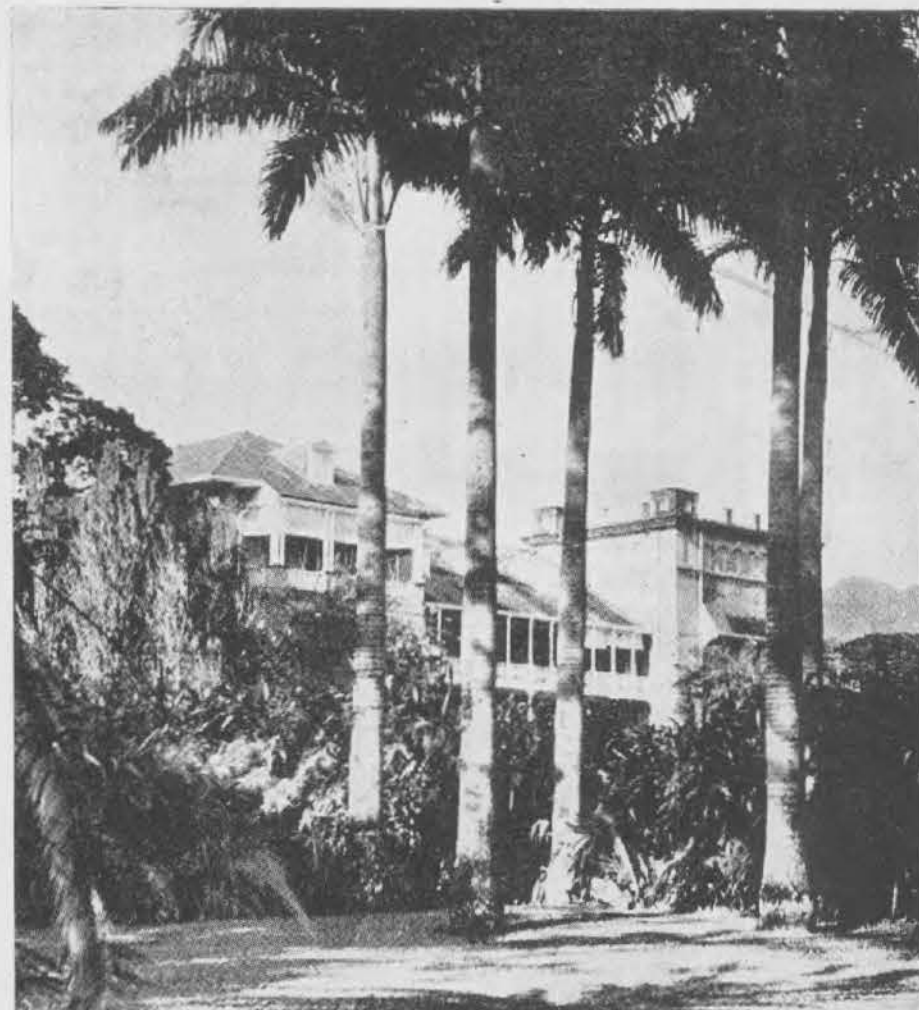
THE GOVERNOR'S MANSION , situated adjacent to the Botanic Gardens, is an imposing structure with lengthy veranda and broad front. Here the Governor dwells amid all the tropic beauty human eyes can see and yet only a few minutes ride from the busiest section of the largest Island city.
