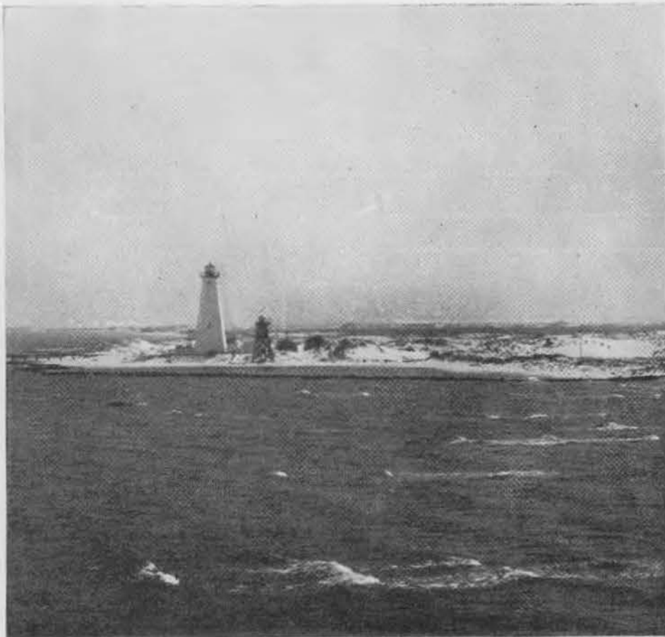
LONE SENTINEL of Mississippi Sound in the Gulf of Mexico is this lighthouse situated on a sandy point of Ship Island. This was one of several islands utilized to train Seabees in the art of amphibious warfare during their residence at A.B.D., Gulfport.
