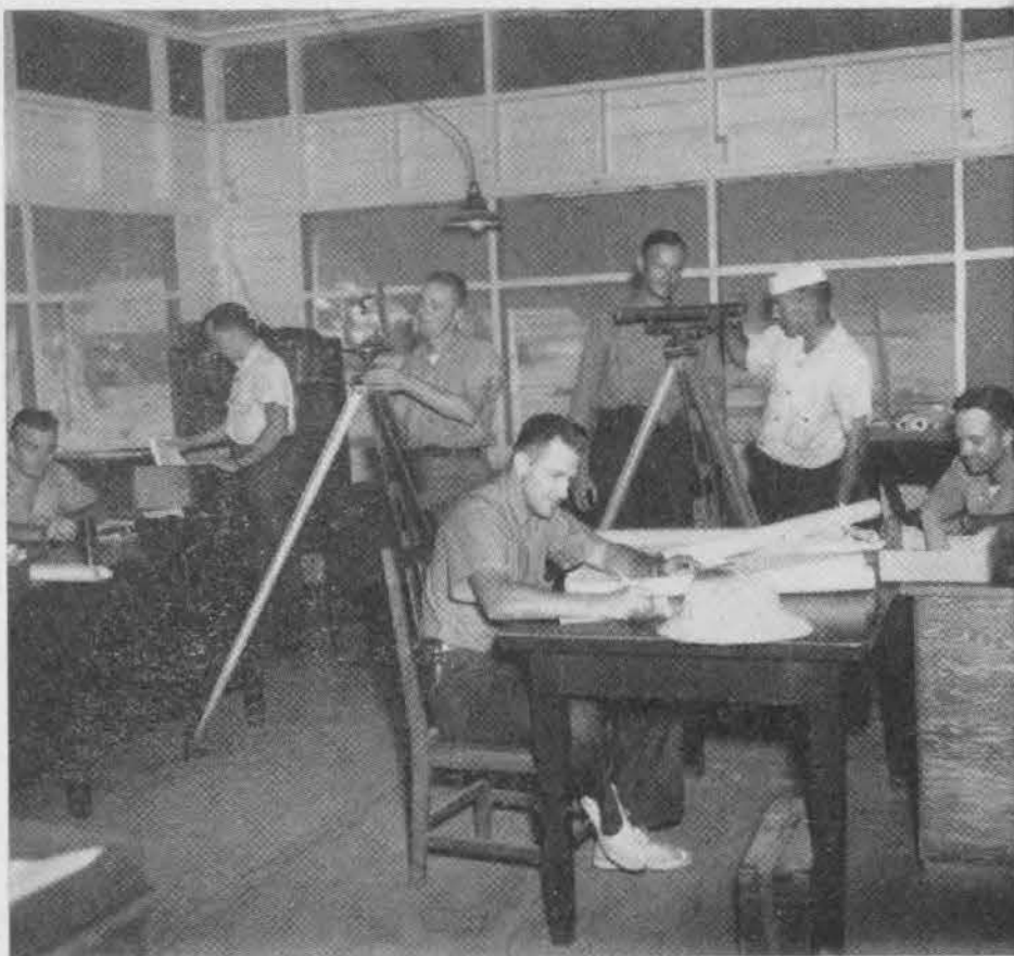
THE FIELD SURVEY OFFICE. The pioneers of any construction job are the surveyors, who with transit, level, rod and chain, lay out sites and submit field notes from which maps, plans, estimates and quantities are platted.
