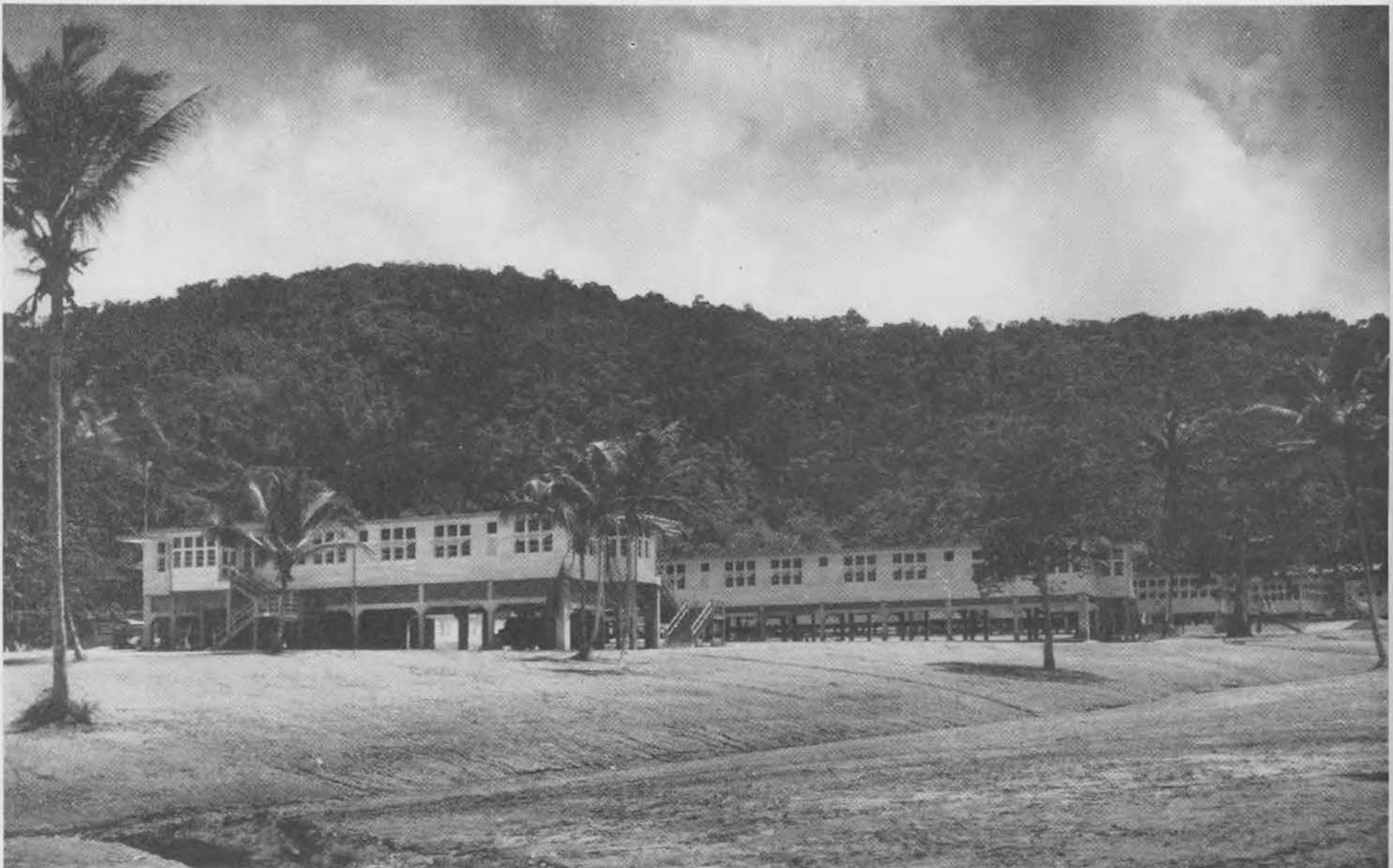
U.S. NAVY HOSPITAL in beautiful Tucker Valley. This project was also taken over by the 33rd Seabees when the work was partially done. It was completed to every detail including landscaping and the paving of access roads. This is probably the most beautiful and best equipped hospital in the Caribbean Area and its location is one to aid the recuperation of convalescent patients.
