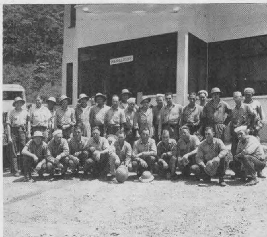
U.S. BULLDOZER. This comfortable spot housed the men who were working on the "town end" of the Road. Formerly some planter's hacienda this spacious stuccoed house nestled in a beautiful valley that even had fruit trees.
