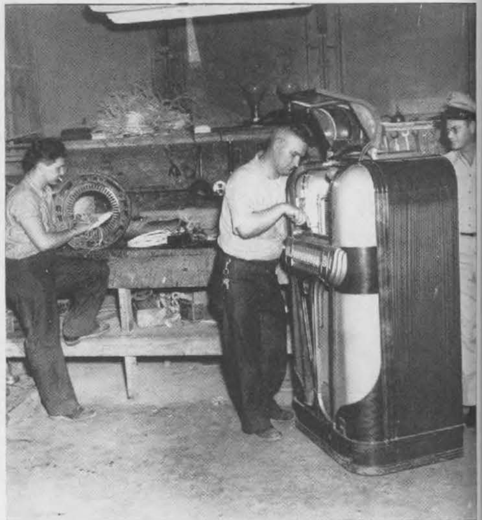
THE ELECTRICAL SHOP. Everyone knows how the electrical gadgets at home used to go "Bloody!" at certain times. They still do in here but our expert repairmen who can fix anything from a giant generator to a juke box, are always on the job.
