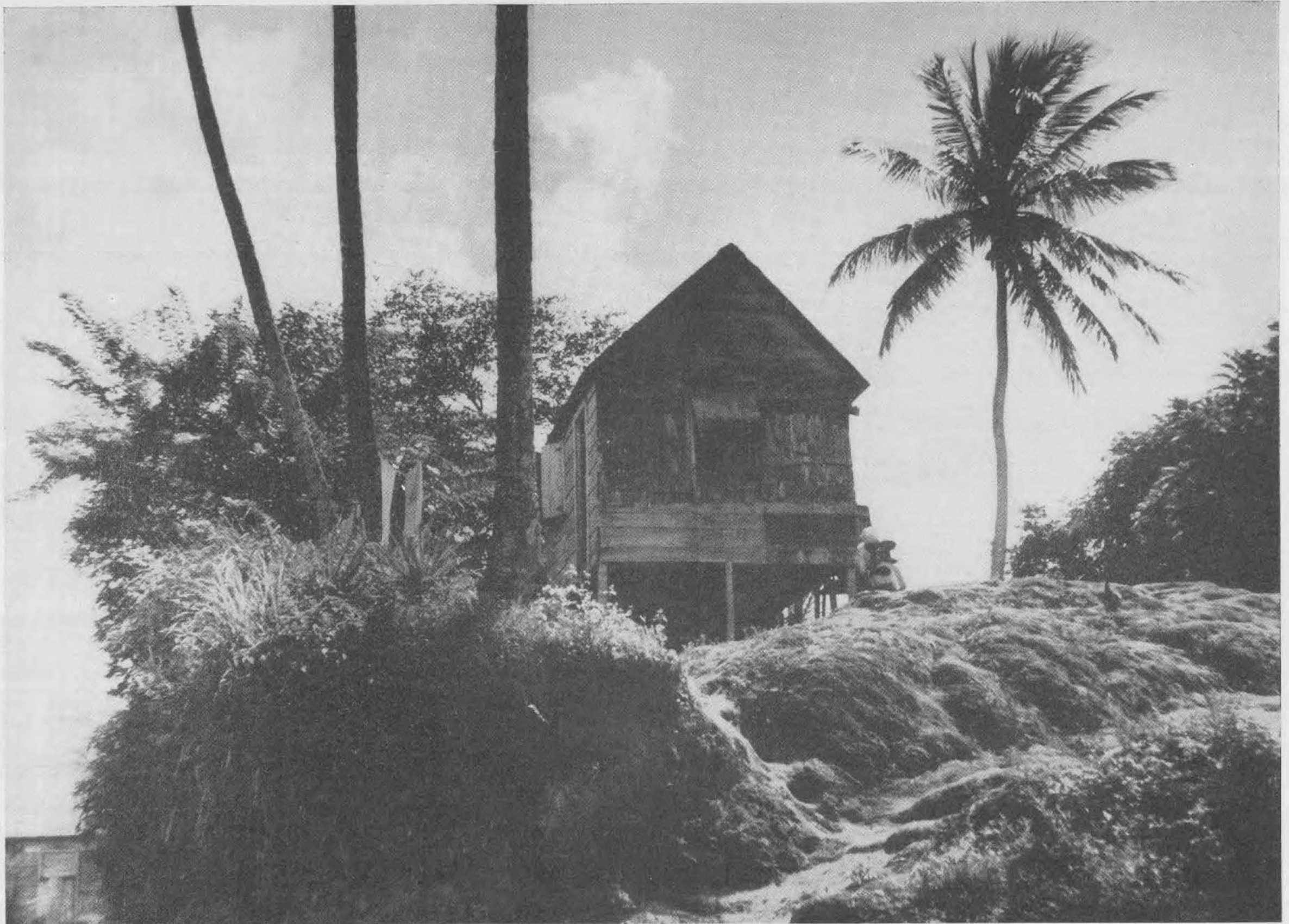
"PICK A SPOT FOR YOUR HOUSE AND SET IT HIGH —then you may be in a position to survey the world and all about you." A native home perched on stilts to protect from reptiles and other ground pests, as well as providing a maximum of comfort from the ever-present tropic heat. Such a house as this may have one large room or a division into two rooms. Sometimes more than one family is crowded together in the one abode as well. Modern conveniences are left to the imagination as the people have neither the money nor the facilities to obtain them. This place may well be labelled as one of the better country homes as the majority are constructed of materials at hand rather than attempting the tedious job of hauling enough lumber overland by oxen and cart from the lumber mill.
