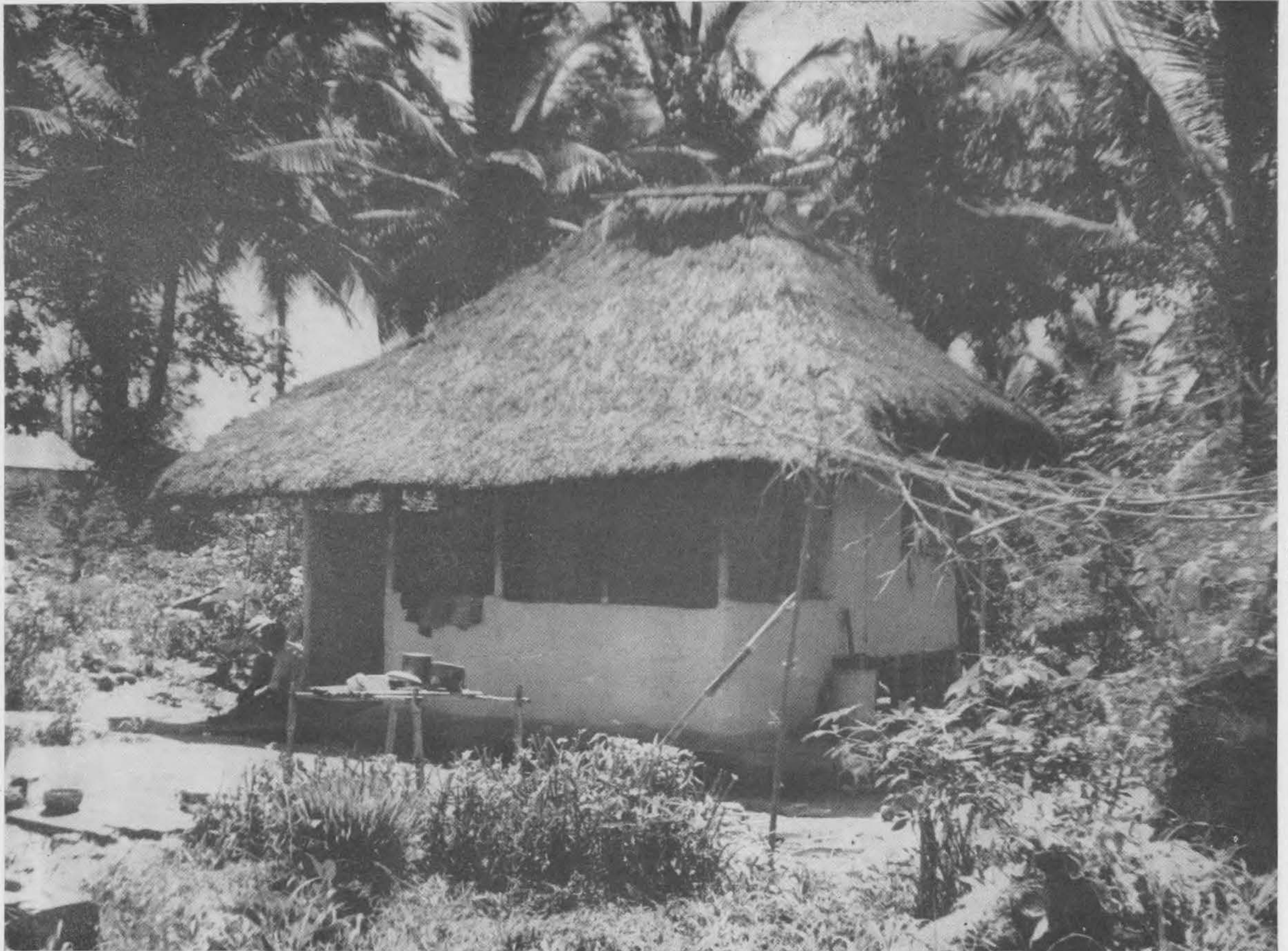
A COUNTRY COTTAGE , constructed with odd twigs, branches, saplings, mud and palm fronds. Affording protection from the sun and rain, this house meets the requirements of its owner without his having had to spend even a modest sum of money. Since the weather is never severe and the temperature varies so little, there is no need for such items as doors or glass windows, thus the people gain a maximum of freedom when moving in and out of doors.
