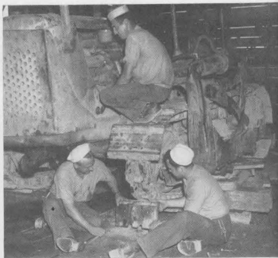
HEAVY EQUIPMENT SHOP. The most hardy units of heavy equipment take a beating in Naval Construction work, especially when operating in rugged and mountainous terrain. When the boys get through working on this battered "Cat," she will return to the wars, almost as good as new.
