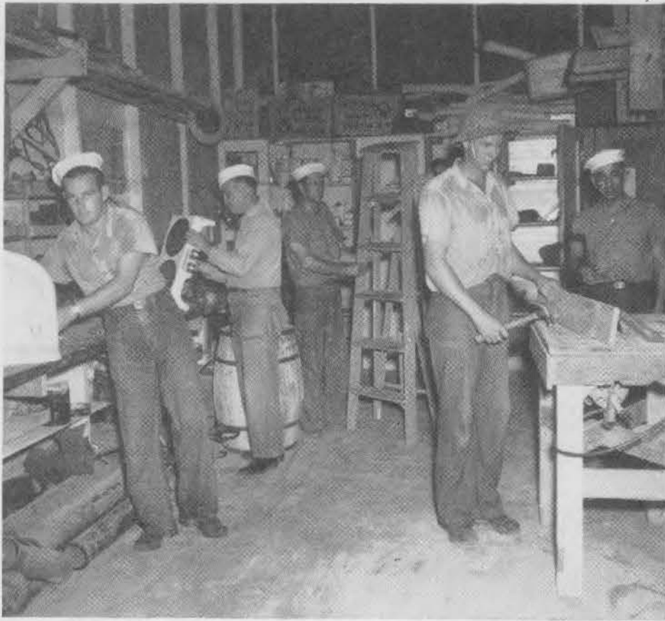
CAMP DETAIL REPAIR SHOP. To the members of the Camp Detail was charged the responsibility for the maintenance of the buildings, grounds, equipment and utilities of the 33rd Battalion Area. They did their job well.
