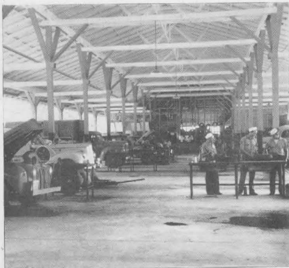
THE MOTOR REPAIR SHOP. Twenty-four hours per day duty does things to rolling stock. Every so often, the toughest of vehicles came to this hospital for treatment and check-up. In this shop, efficient mechanics and repair-men made speedy adjustments in order to keep everything rolling.
